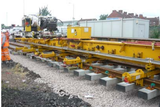
Kirow 250 relaying S&C at Worksop
